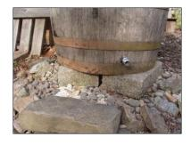
Prepare a level area to place the barrel. Some stone or cinder blocks work well
