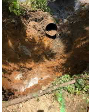
Discharge During Construction
