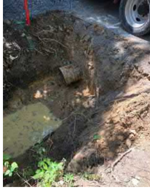
Discharge During Construction
